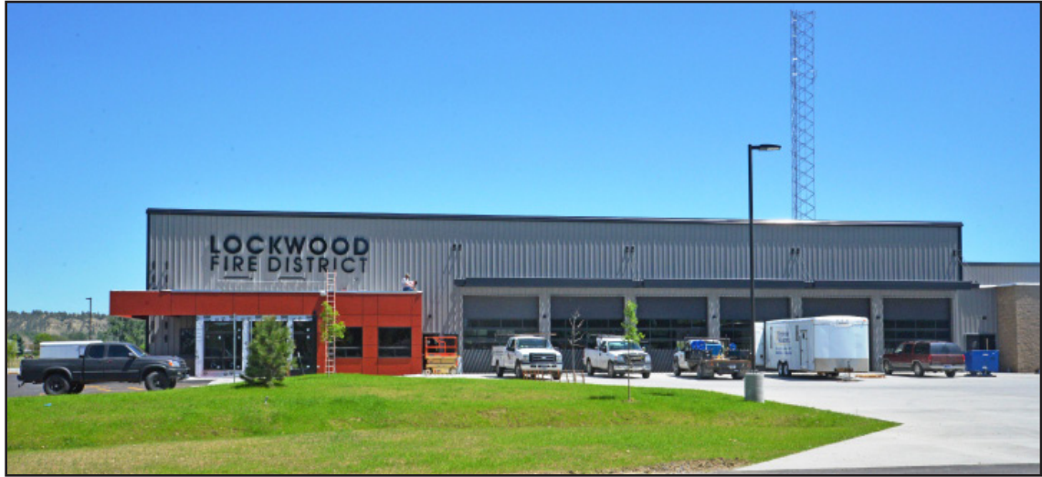
The Lockwood Fire District's new station is nearing completion and should be ready to occupy later this summer. The project is well under budget, allowing fire officials to consider options such as additional electrical outlets. (Jonathan McNiven photo)
